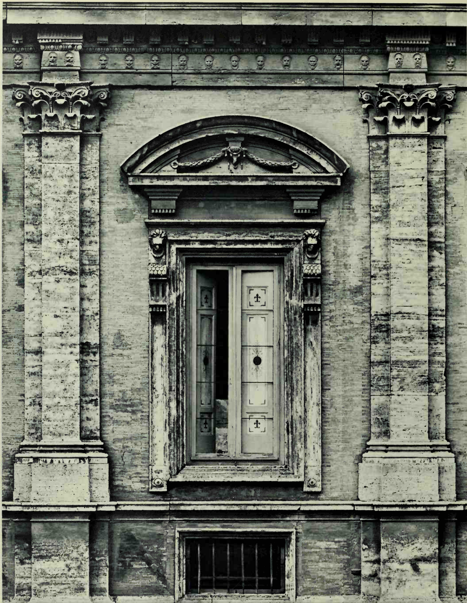
260. PALAZZO FARNESE. Window in the upper storey of the courtyard. About 1550
