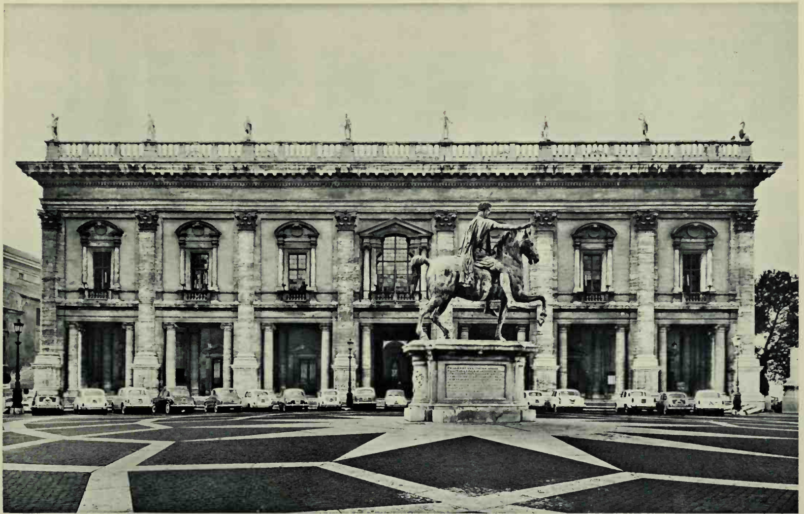
254. PALAZZO DEI CONSERVATORI, ROME. Planned by Michelangelo in 1546, finished after his death
